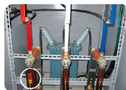
Abnormal Temperature Detection for High-Voltage Fuse Overload
