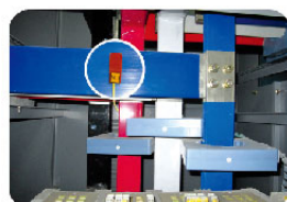
Abnormal Temperature Detection for Power Bus Bar
