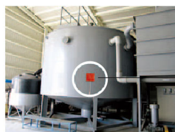
Temperature Sensing of Large-scale Storage Tank (Connection Example)
