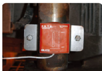
Abnormal temperature detection for power plant, cogeneration plant, heat recycling pipe, and ash ejectors (Example in Formosa Plastics)
