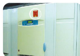
Temperature Sensing for UPS Machine Room
