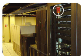
Abonormal Temperature Detection for Communication Machine Room
