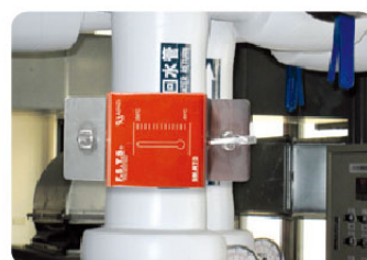
Abnormal temperature detection for the return-loop water used in the cooling water for air conditioners
