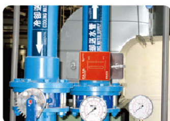
Abnormal temperature detection for the cooling water used in the chiller for air conditioners
