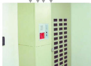
Centralized Temperature Monitoring Panel (RS485)
