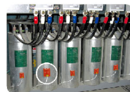
Abnormal Temperature Detection for Capacitor Cabinet
