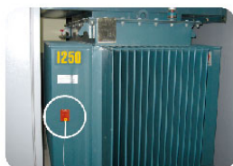
Abnormal Temperature Detection for Transformers
