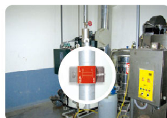
Abnormal temperature detection for steam pipes (Example in Shangcun Chemical)
