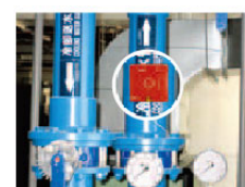
Abnormal temperature detection for air conditioner pipe (Installation Example in Shangcun Chemical)
